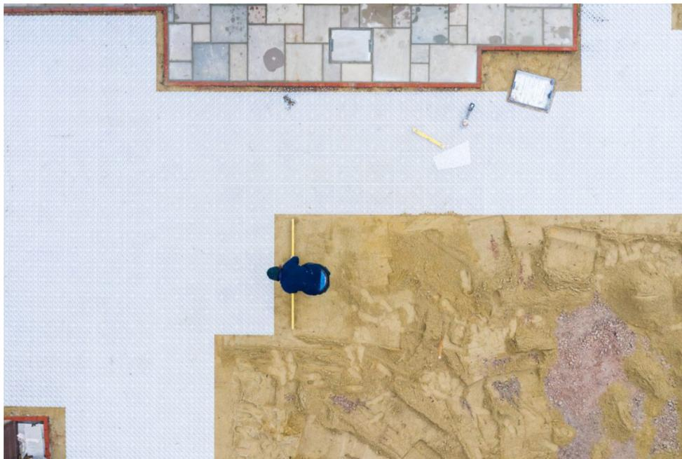
Gravelrings sets itself apart by being a one-piece moulded system. The mesh-backed base anchors the grid into the ground, preventing gravel from sinking the system, as well as from lifting up the panels and exposing them. The mesh base also allows the free-flow of air throughout the system, preventing the build-up of silts and fines that encourage pesky weed growth, thereby reducing maintenance requirements for the client.
