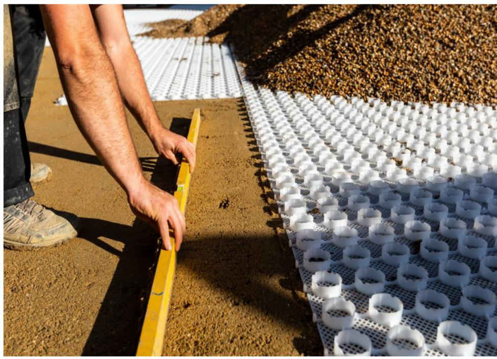
The added benefits of using Graveledge alongside Gravelrings does not come at the expense of a tricky installation. Graveledge edging can simply be installed around the perimeter of the gravel driveway with a dry fix installation, meaning no concrete is required. Even better, Graveledge is flexible enough to create curves or straight lines by hand, making installation simple and seamless.
